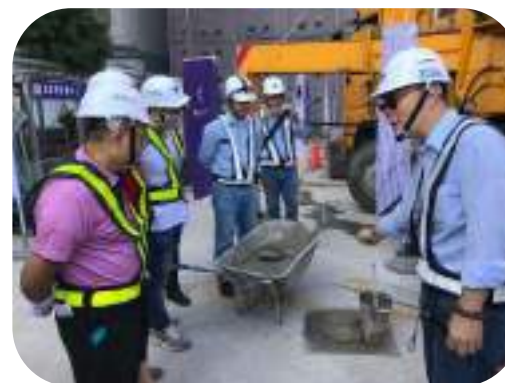
混凝土坍度實驗
